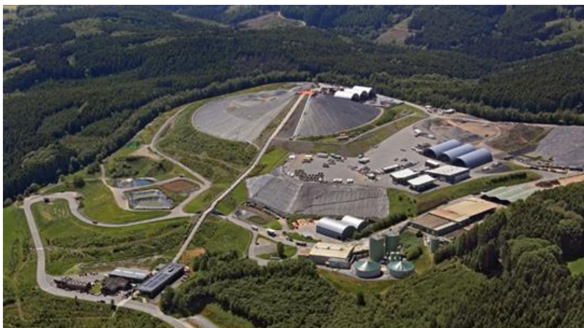
Aerial view of disposal centre Leppe, location of :metabolon (Source: BAV)
